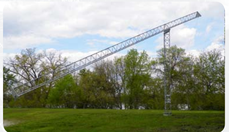
60' ROHN 55FK shown in lowered position
